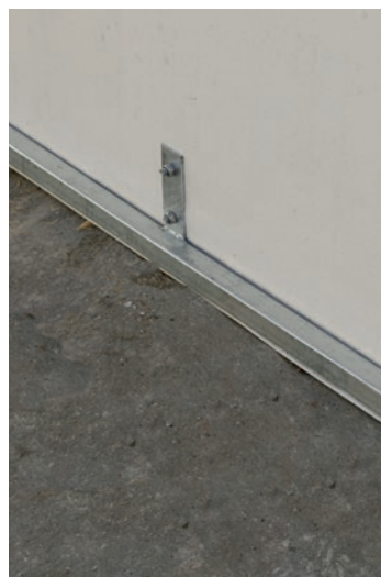
The reinforcing frame gives the house additional stability
