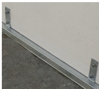
The reinforcing frame gives the house additional stability
